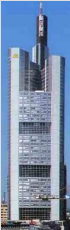
Commerzbank Frankfurt 30 elevators
