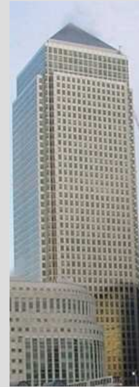
Canary Wharf London 36 elevators
