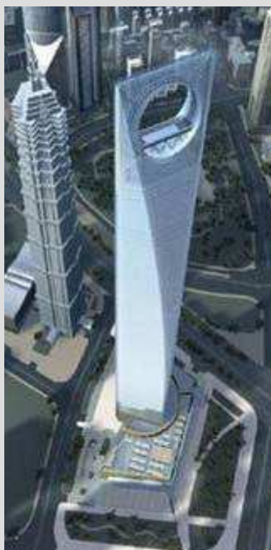
Shanghai World Financial Centre 92 elevators
