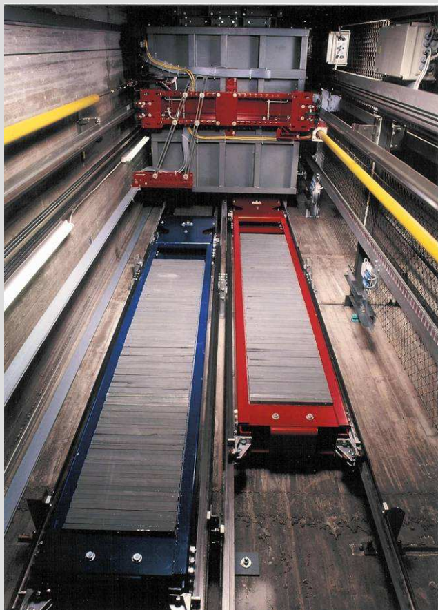
Upper car with both counterweights
