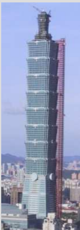
Financial Center Taipeh 63 elevators
